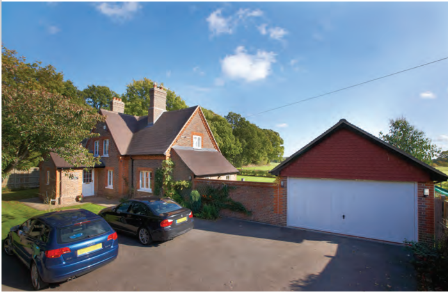
Two-storey extension, with new front porch linked to new garage.
