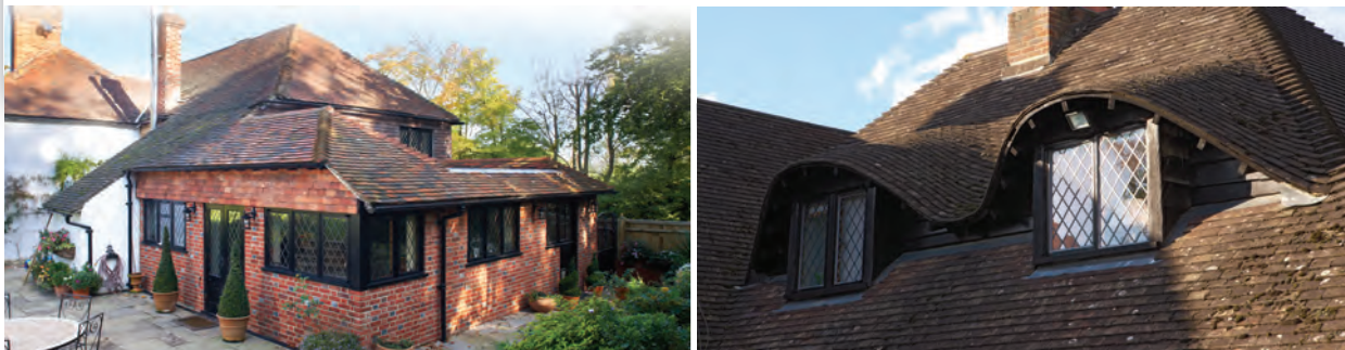
A single-storey extension providing larger kitchen, utility room, dining area plus feature patio and retaining walls. Eye brow windows with oak joinery.
